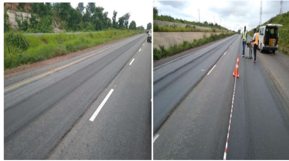
Figure 1: Rutted sections of Abuja-Lokoja highway
